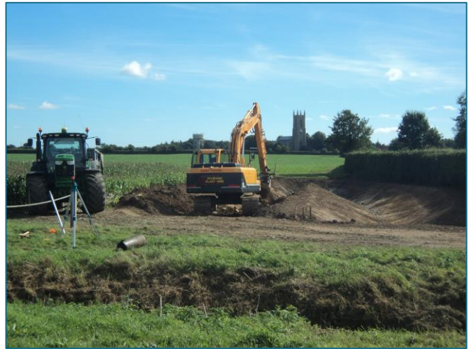
Figure 5. Construction of silt trap 1 (SUD 1) at Salle. Credit: Norfolk Rivers Internal Drainage Board.
