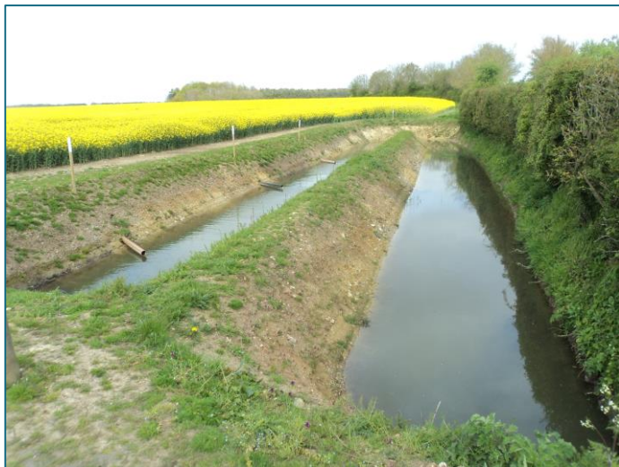
Figure 6. Silt trap (SUD 2) complete and draining water. Credit: Norfolk Rivers Internal Drainage Board.
