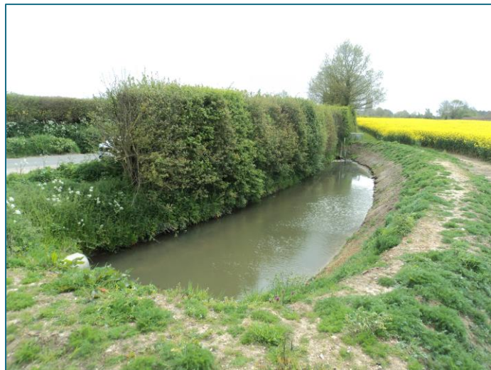
Figure 7. Silt trap (SUD 3) complete and capturing run-off. Credit: Norfolk Rivers Internal Drainage Board.
