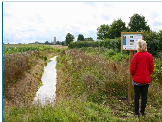
Figure 9. The interpretation board has been installed to explain the purpose of the silt traps to the public.
